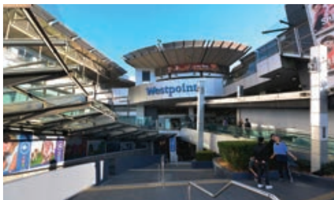
CENTRE COMMERCIAL WESTPOINT - BLACKTOWN - AUSTRALIE
