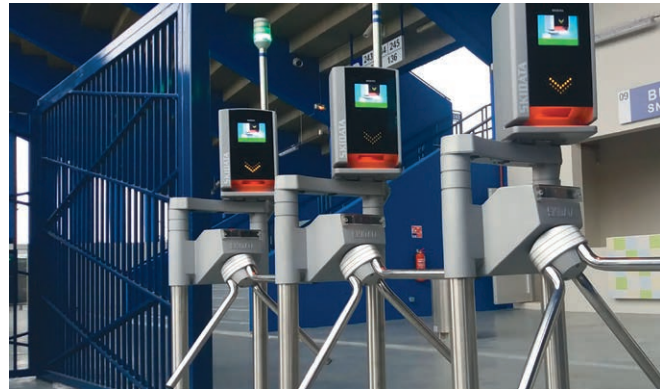
FRANCEVILLE STADIUM – FRANCEVILLE – GABON
