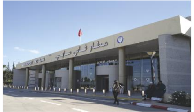
FÈS-SAÏSS AIRPORT - MOROCCO
