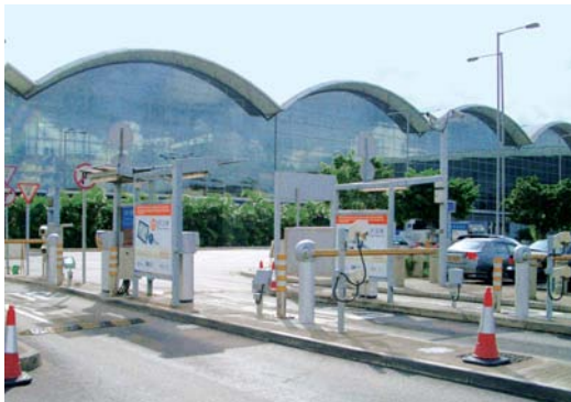
Hong Kong Airport car park
